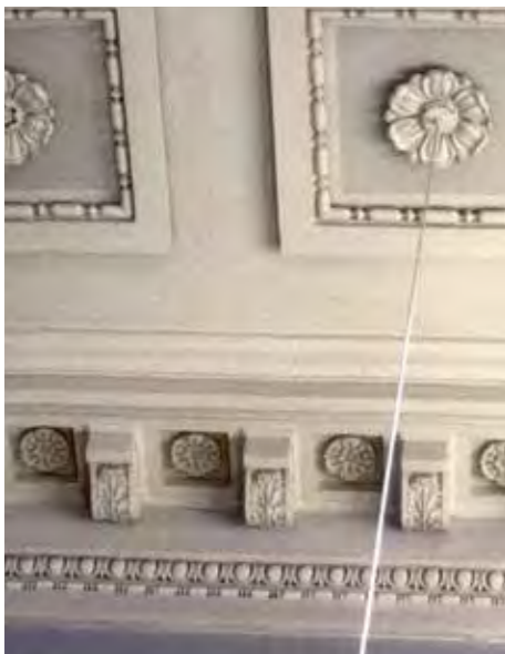
Detail of the stucco ceiling in the Ceremonial Hall at Charlottenborg.
