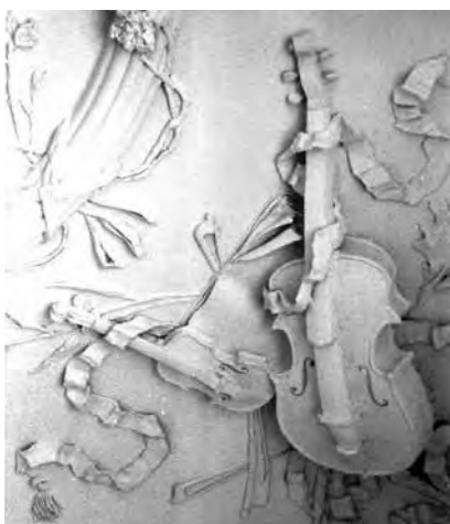
On the somewhat rough cores, we modelled the figures up with the same mixture of lime-mortar and plaster, mixed up in the form of a weak plaster; we didn't apply this mixture until it had the consistency of whipped cream.
